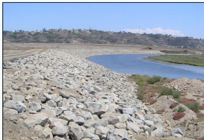
Rock berm protection along river bend in Area 3.
