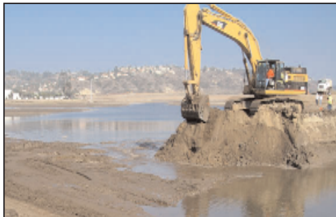
The excavator at work to break down dirt berm.
