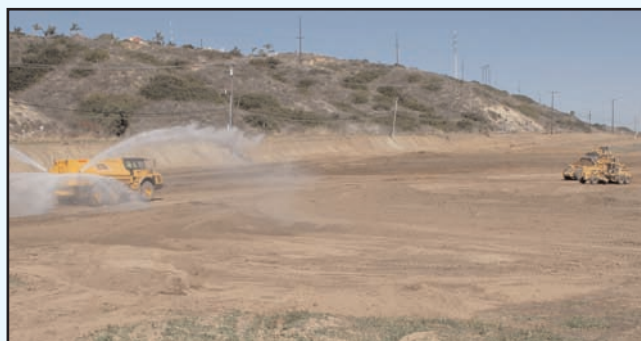
Water Truck Minimizing Dust in Area 3
