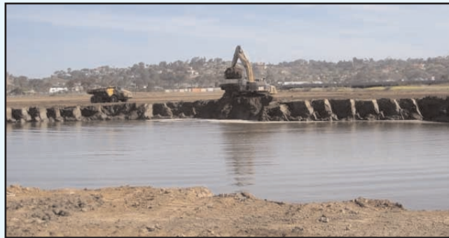
Excavation Work in Area 2A
