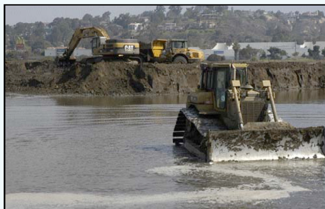
Dozer cutting grade in water in Area 3, north of river
