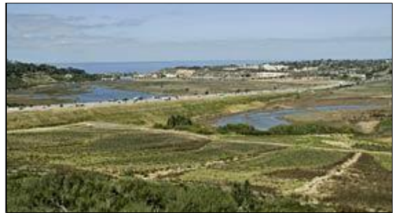
DON KOHLBAUER / Union-Tribune The San Dieguito Wetland Restoration Project will cost $86 million, and its expected launch date is late summer or early fall. It should take about three years to complete. The project involves 440 acres on both sides of I-5.
