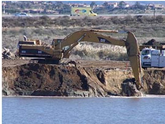
Crews use construction equipment to excavate dirt Jan. 15 from the W-1 wetland module of the San Dieguito Lagoon restoration. (Photo by Scott Landheer)
